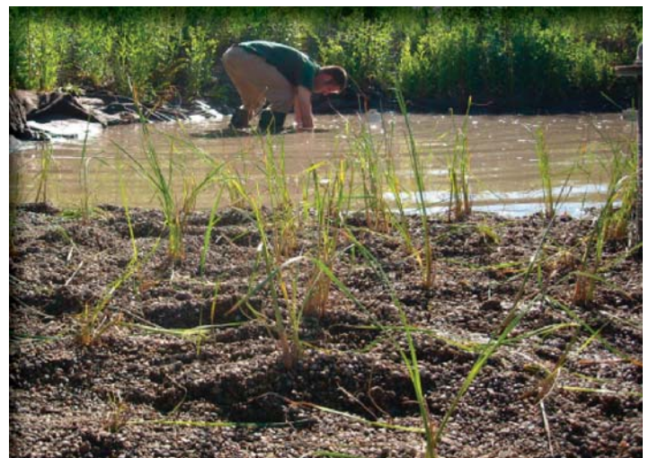
Wetland Treatment Cell Plug Installation
